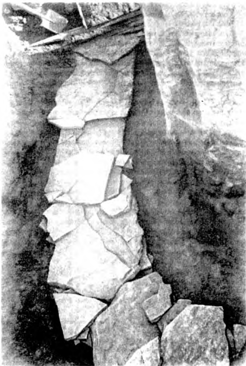
Figure 31. Channel-smoke duct under the floor of the palace. Channel was tightly sealed, lined on both sides and at the top by perfectly fitting stone tiles (photo, 1945)
